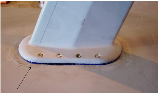
Figure 6-6. Typical Gel Squeeze-Out Around Perimeter of Antenna
